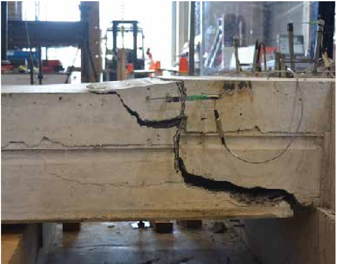
Damaged hollowcore floor after testing. Photo: The University of Auckland.
