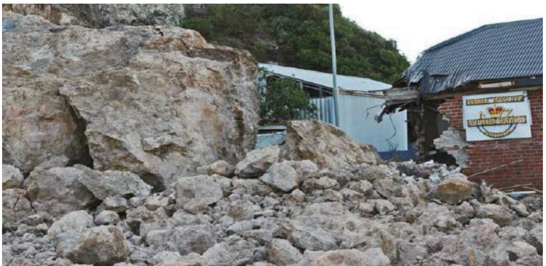
Figure 2-51: Dislodged boulders near the RSA clubrooms following the Feb 2011 Christchurch earthquake. Photo: Margaret Low, GNS Science.
