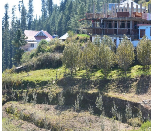
Fig. 12: Terraced slope stabilization with vegetated surface
