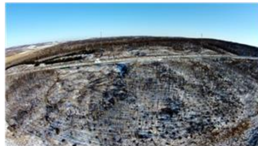
Figure 12. View of the K179+600 landslide
