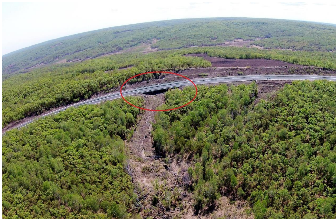
Figure 28. Replacing the road section with bridge
