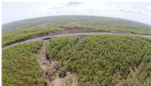
Figure 11. View of K178+530 landslide
