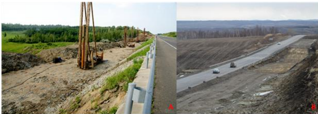
Figure 27.Using hot gravel piles for Permafrost Foundation treatment
