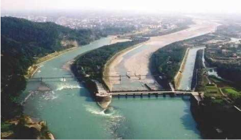
Dujiangyan Irrigation System
