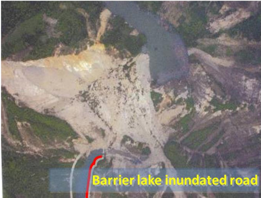
Landslides buried subgrade
