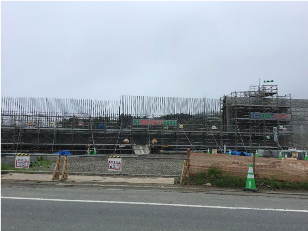
Figure 4. Seawall under construction, Ogatsu town, Miyagi (taken by author in July 2019)
